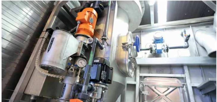
treatment, biological treatment and sludge dewatering. Furthermore, the Box4Water is equipped with a touch screen control panel with remote monitoring and control, allowing visualisation and operation of the plant without being present on site. The Box4Water, which can treat up to 120 m<sup>3</sup>/day (600 population equivalent), in most cases avoids the use of chemicals and meets international and European highest requirements for direct discharge.
